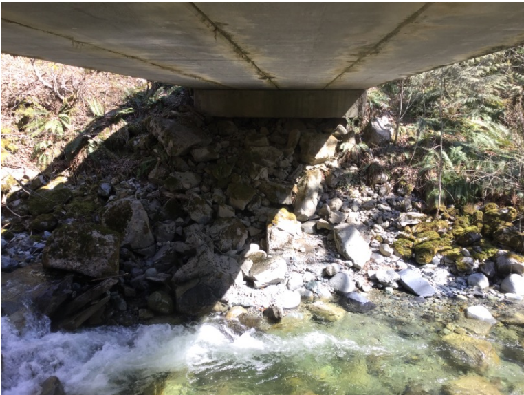
Left Bank Abutment when facing downstream
