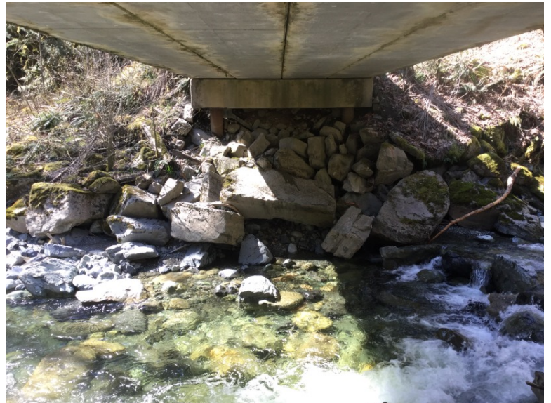
Right Bank Abutment when facing downstream
