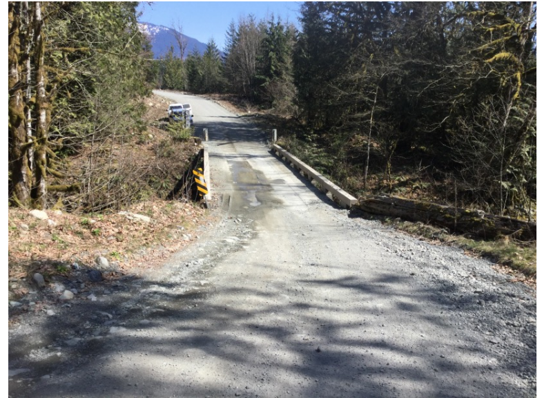
Right Bank Abutment when facing downstream
